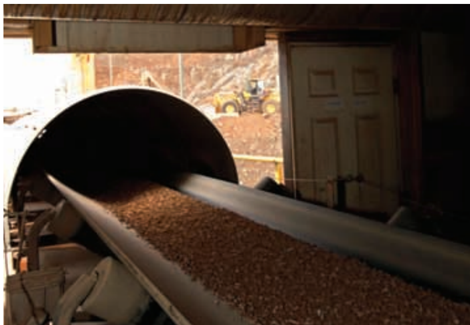
Jim Sims, vice president of corporate communications for Molycorp, top, shows the vats that hold solvents for extracting elements at the Mountain Pass rare-earth facility in California's Mojave Desert. Center, Jeff Adams, control room operator for the mill. Above, crushed rock is conveyed into the mill where it will be turned to powder for further processing. JOHN GURZINSKI
